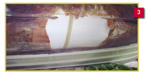
Using matting and a biaxial stitchmat, the laminate is built back up as close as possible to the boat's original lay-up. Because of the way the side of the boat was torn open, it was possible to count the number and type of the laminations.
