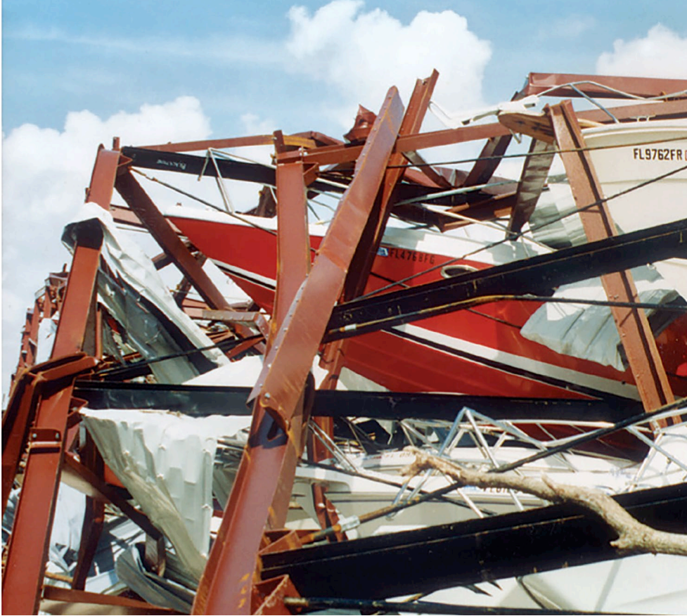
High-rise storage racks can be toppled by a storm's high winds. Especially if your boat is in an older building, which is likely to have been built to less stringent standards, consider putting it on a trailer and moving it further inland.
